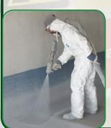
together with the technical team from VIP, recommended VIP Quickspray Industrial-Slow, a polyurea based coating system that cures and hardens rapidly, but slower than some of VIP polyurea systems, in order to allow the surface profile to be obtained / built-up as required - textured and slip resistant or smooth.
